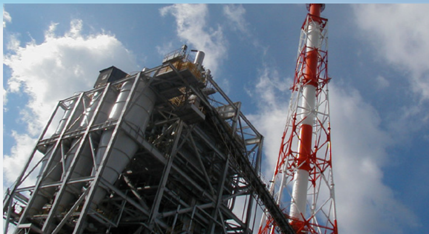
This on-site power generation facility is being renewed
