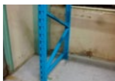
Some racks had no anchor bolts and were prone to tipping over. We checked and up-graded all racks, fixing them with anchor bolts
