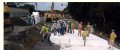
Also used to widen roads
