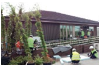
Participants had to complete construction of the eco-houses by a strict deadline
