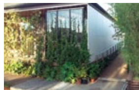
The green curtain cools the structure
