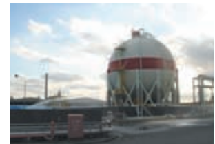
Training in tank water spraying
