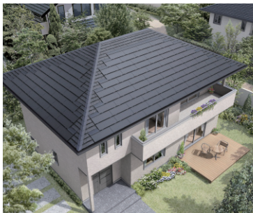
Photovoltaic modules designed specifically for decorative slate tiles
