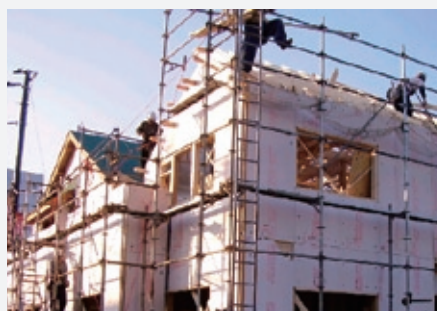
Using Kanelite Foam as insulation helps cut electricity consumption from air conditioning.
