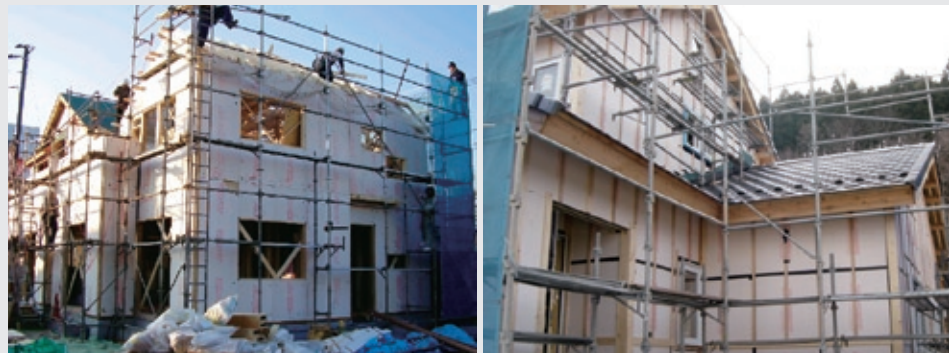
Using Kanelite Foam as insulation helps cut electricity consumption from air conditioning.
