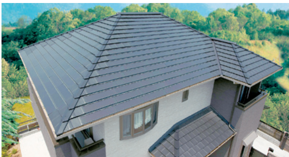
Form meets function: Roof-integrated photovoltaic modules
