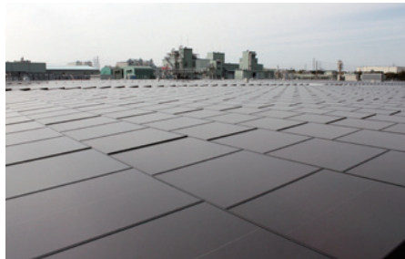
Megasolar system in the west area of Kashima Plant
