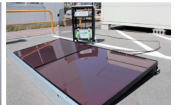
Solar power generation system
