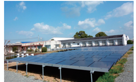
Kyushu Kanelite Co., Ltd. installed ground and roof panels
