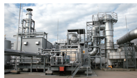
Deodorizing furnace waste heat recovery steam boiler
