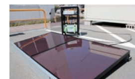
Solar power generation system
