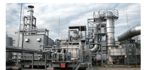
Deodorizing furnace waste heat recovery steam boiler
