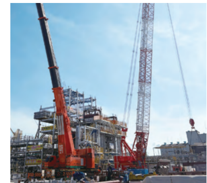
A new gas turbine cogeneration system being installed
