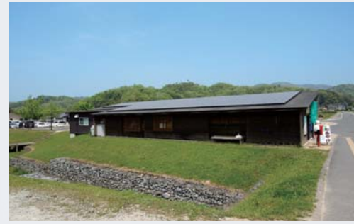
A rest house at the stork preserve donated by the Group featuring a roof mounted with solar panels
