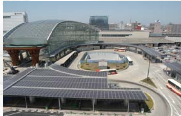
See-through photovoltaic modules installed at a bus terminal outside Kanazawa Station
