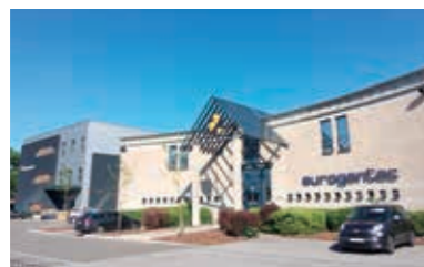
Biopharmaceutical contract development and manufacturing building of Kaneka Eurogentec
