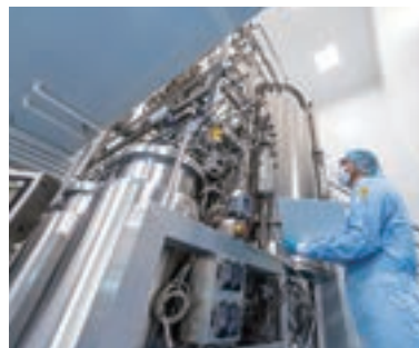
Biopharmaceutical manufacturing facility
