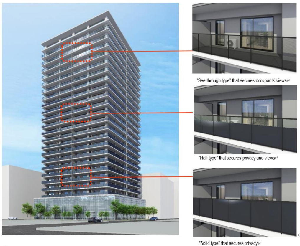
Figure 1: Image of "T-Green Multi Solar" glass balustrades installed on ultra-high-rise condominium
