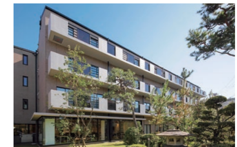
Kaneka “Dreamology” Center with low-reflective solar cells installed on walls and handrails equipped with thin-layer see-through solar cells that transmit light
